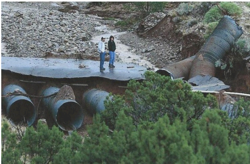
Flood damage on Huertas Creek in Placitas, NM (2006)
