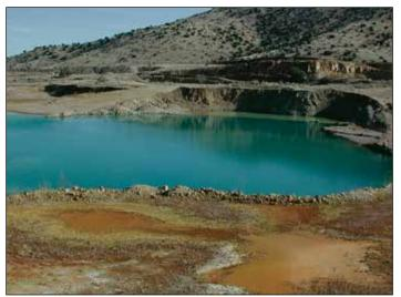
Photo courtesy Gila Resources Information Project The pit where the former Copper Flat Mine hit groundwater and water filled the pit.
