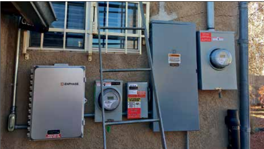
Solar costs have gone down more than 70% since 2011. Carol Chamberland's new system, left to right: micro-inverter control panel, R.E.C. meter, Photovoltaic system disconnect, home electrical panel and PNM meter.
