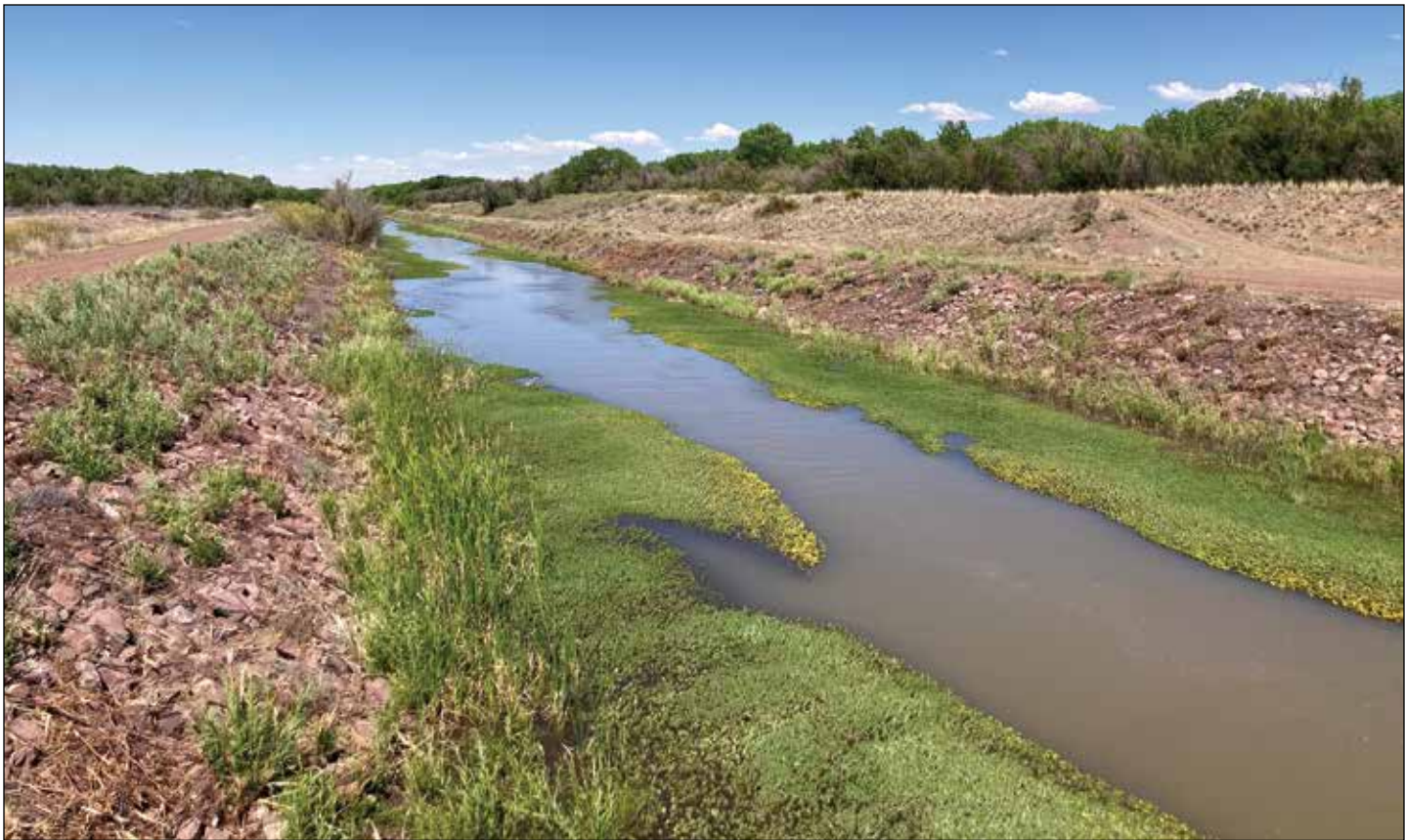
The Low-Flow Conveyance Channel was built in the 1950s to get water to Texas and avoid the Rio Grande. Sedimentation forced its abandonment in the 1980s, but it might be seeing a revival.
