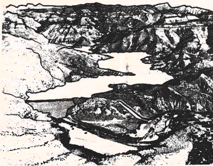
Photo courtesy of the Bureau of Reclamation
